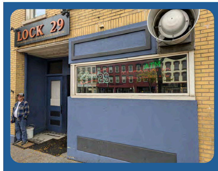
2024 - Current view of 138 E Main St. Note all the windows on the 3 rd floor are boarded up, front, sides and back. Third floor is unusable, and currently dark and vacanr. Hard to see in this picture, but mortar joints are heavily deteriorated, leaving spots for bees to nest and weather to enter. 1 st -floor glass and entry are in poor repair, and detract from the building aesthetics
